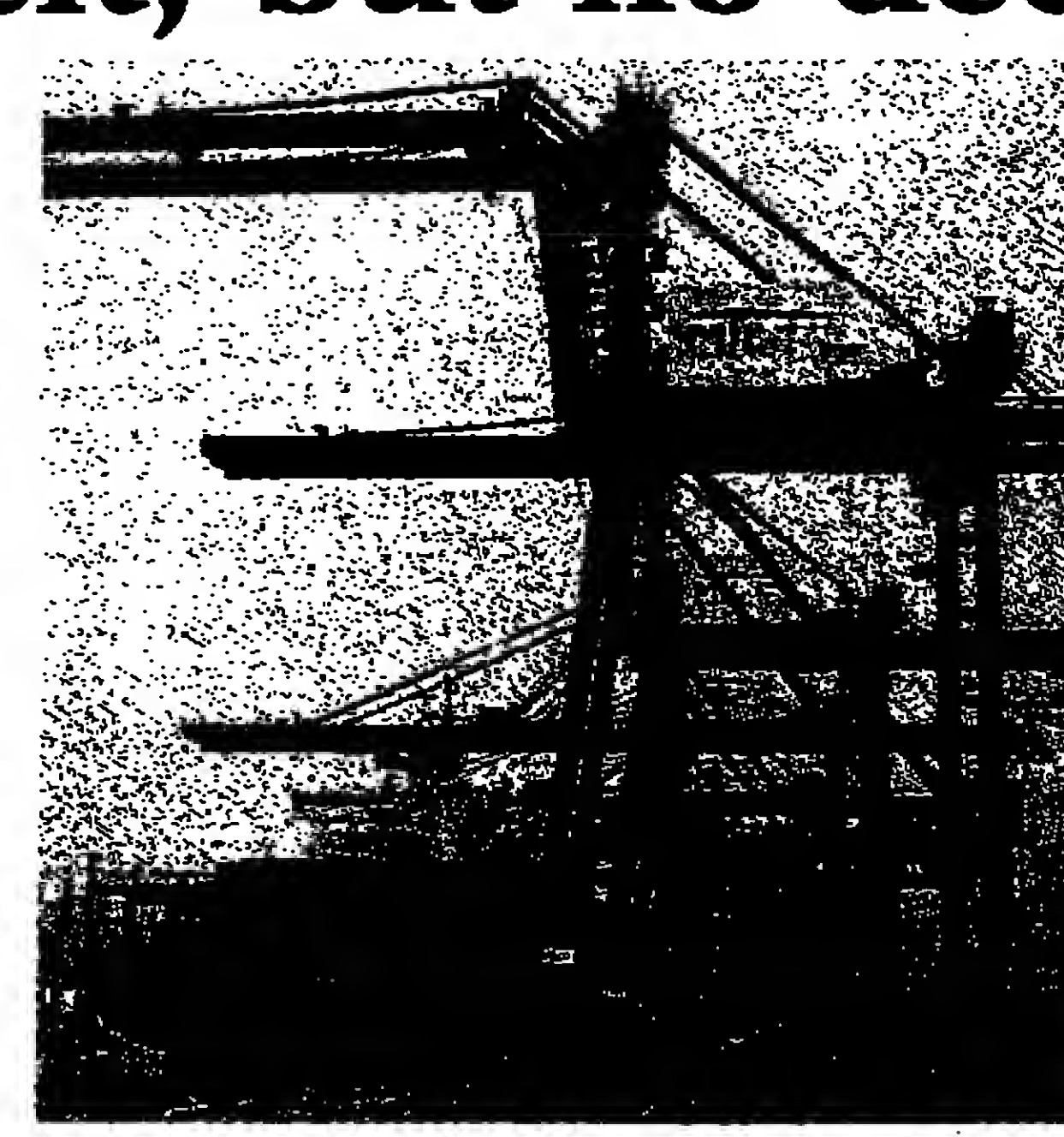
Terminal progress: the world's biggest container port is expanding
